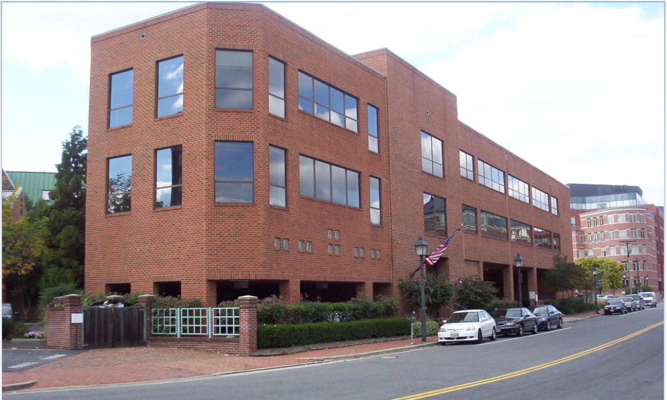
NSBE World Headquarters Building – Alexandria, VA
